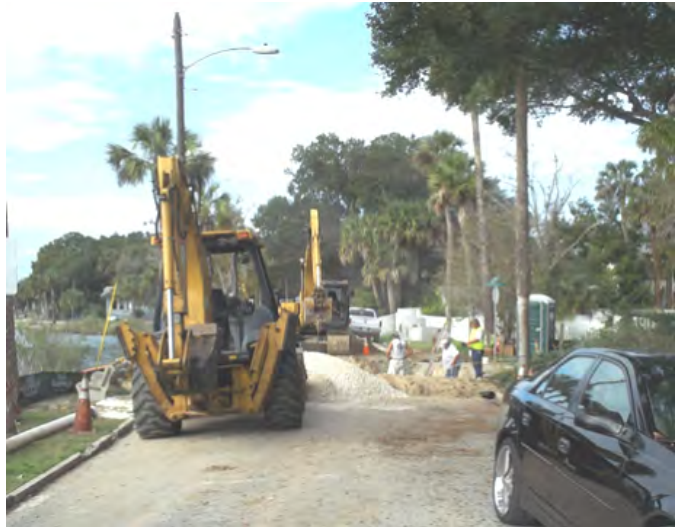
Crews prepare site for installation of new drainage system.
